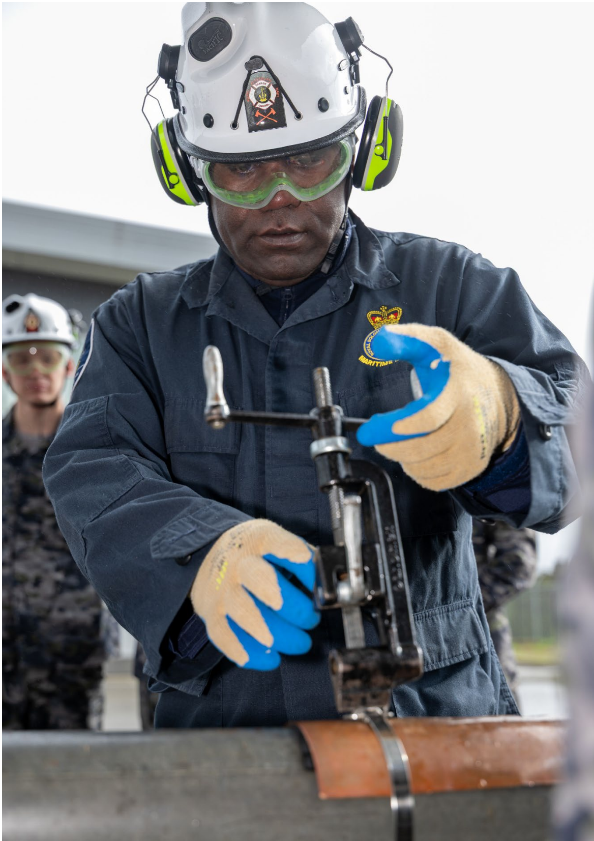
Caption: Police Constable Justin Apa conducts a pipe repair during the leak stop training stand at the School of Ships Safety and Survivability.
